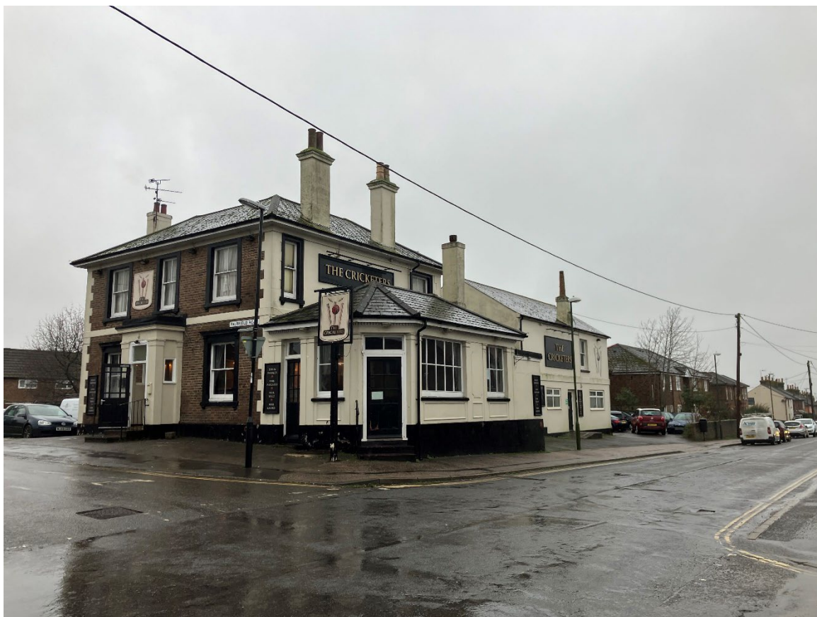
Photos of premises from Junction West Street and Fairfield Road
